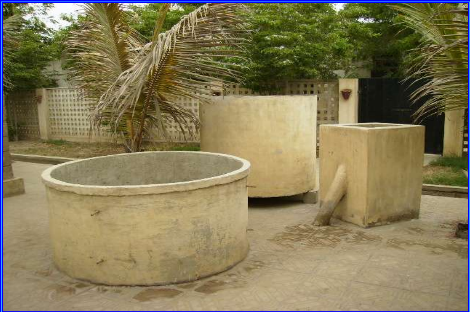
Ferrocement Bio Gas Plant
