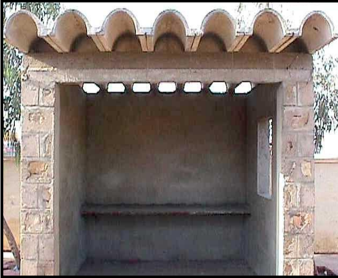
FERROCEMENT BARREL SHELL ROOFING SYSTEM
